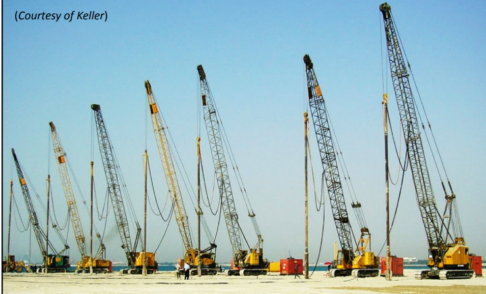
Vibro Compaction (VC) typical treatment depth ~ 8 – 15m (50m)
