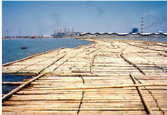
Utilization of Bamboo Mattress for Coastal Embankment at Tambaklorok - Semarang
