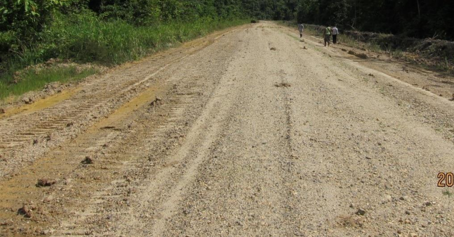
Road after construction
