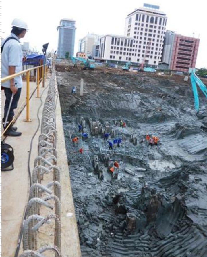
Excavation in Jakarta Marine Clay
